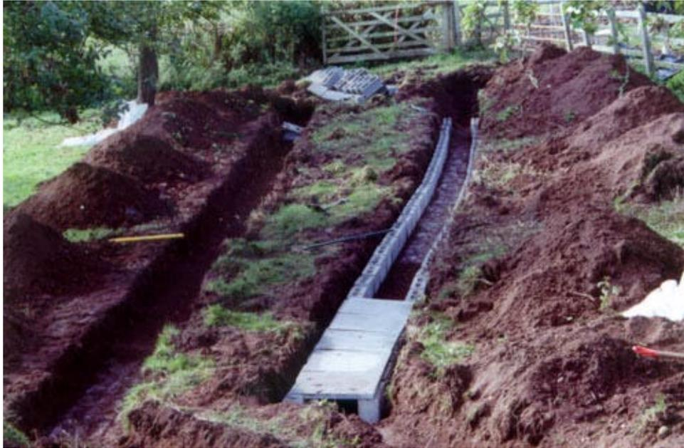
Figure 1 this system for a house has two parallel trenches. Both have been excavated and the bases have been laid so the first 6 metres fall at 1:20. The blocks have been laid with a gap of about 30 mm between them and the slabs lay on the top. Please note that the base of the trench ahead of the slabs has been raked to avoid smearing and compaction.
