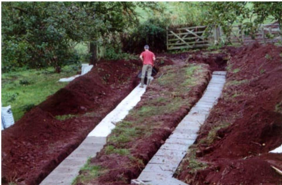
Figure 2. The trenches are now both covered by the slabs and the geotextile is laid on the top.
