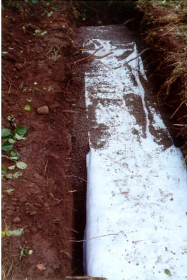
Figure 3 Clean stone – 20mm average – is laid in the gap outside the blocks to the level of the slab. Earth and turf is laid over the blocks to bring the level up to that of the surrounding soil. Note the roots showing that the system has been created in the topsoil. The size of the void greatly reduces any danger of blockage by roots.
